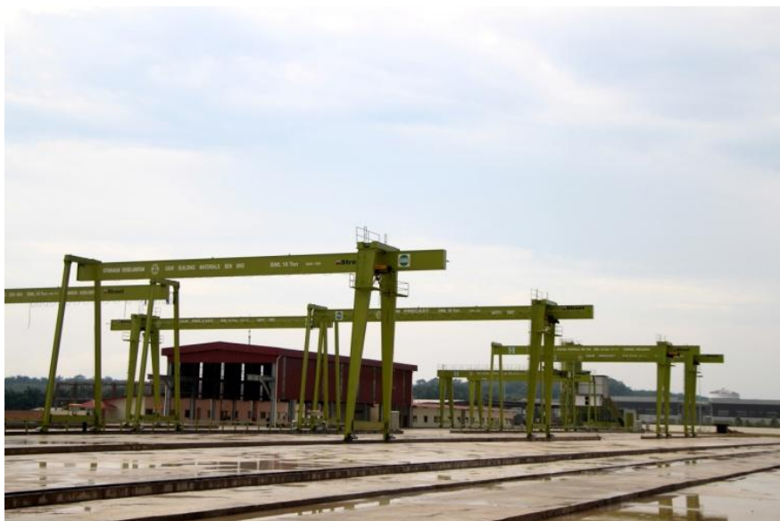
The 47,000 sqm Iskandar Precast Plant has an annual production capacity of 75,000 m 3 .
